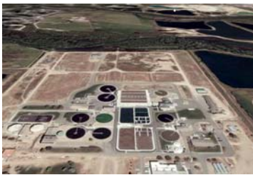
Aerial view of West Boise Wastewater Treatment Plant, courtesy of City of Boise.
